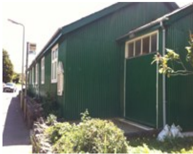
Flooded - to be demolished
